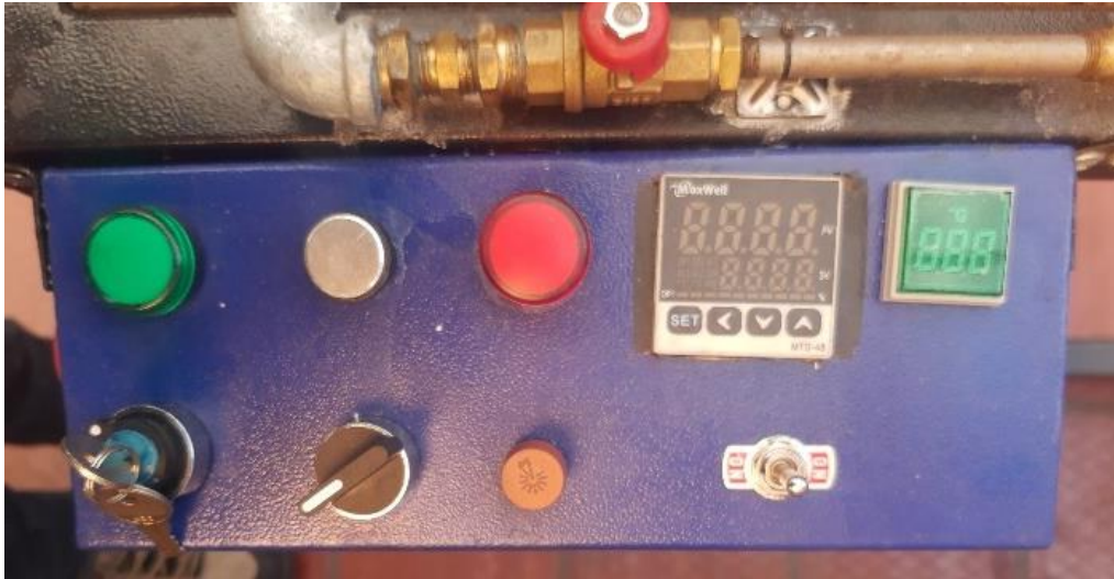
Figura 52. Panel de control
